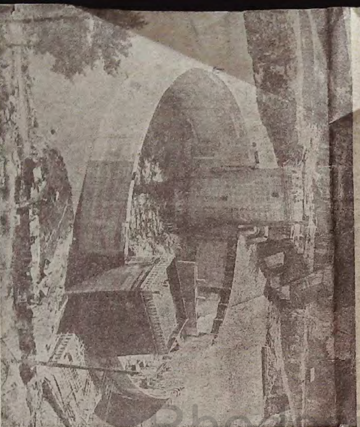
FLOODWATERS race round the thin concrete walls of the Kariba coffer dam. When the picture was taken late yesterday afternoon only 7 ft. of the coffer dam stood above the flooded Zambezi, which is already level above last year's record level. Workmen can be seen battling to raise the bulk of the upstream wall with a barrage of sandbags, reinforced with steel rods. In contrast, the smaller picture, taken a week ago, shows the water well down and work on the four stations of the main wall going ahead.
