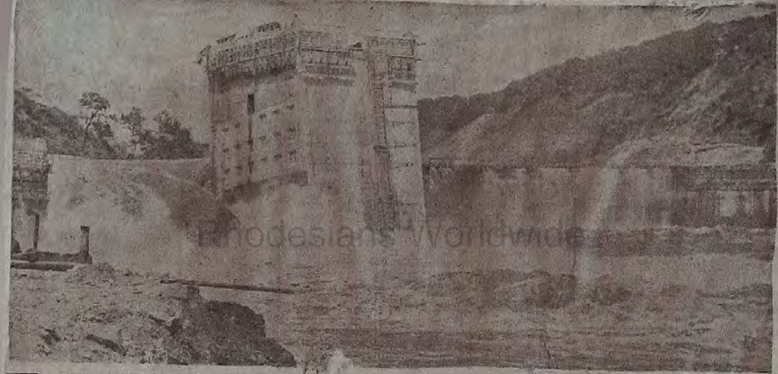
T HE waters of the rising Zambesi finally top the upstream wall of the big circular cofferdam at Kariba, in spite of it being raised a further 12 feet. On the left the river roars through the blocks of the main dam wall.
