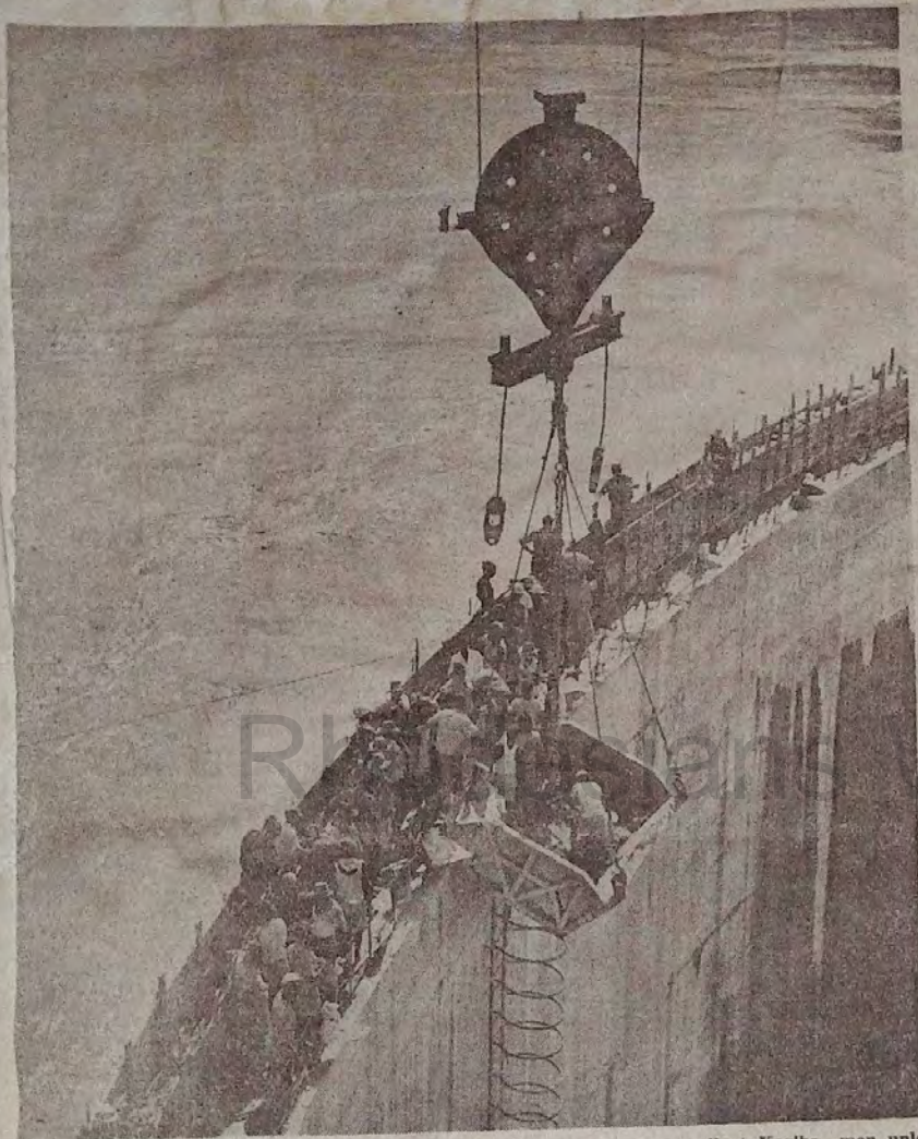
LEFT: From the top of the south bank block of the main dam wall at Kariba—men unloading sandbags from a Blondin bucket to pack on to the upstream edge of the cofferdam. Right: The view from the south as the Zambesi, built up by the cofferdam, rages through the blocks of the main dam wall.
