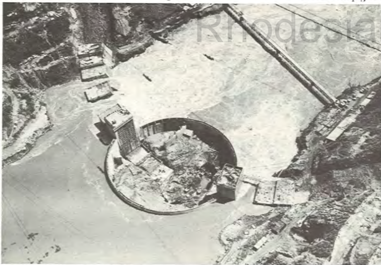
February 1958 and the flood-waters were rising (see page 39). The coffer dam technique provided areas of dry river-bed to make construction work possible.
