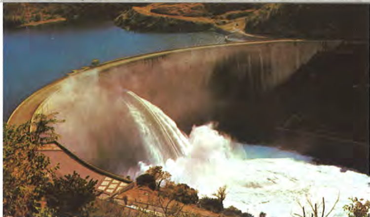
Above: The 128-metre-high Kariba Dam, opened in 1960, holds back a lake with an area of 5 000 square kilometres. The centre of the dam is the border between Rhodesia and Zambia.
