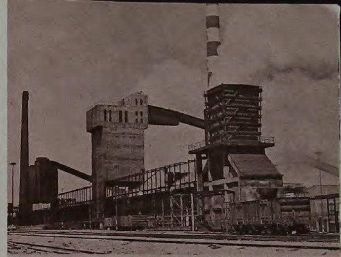
Risco's battery of coke ovens which use coal from the vast Wankie coalfields to produce the coke which is vital to the iron-making process.
