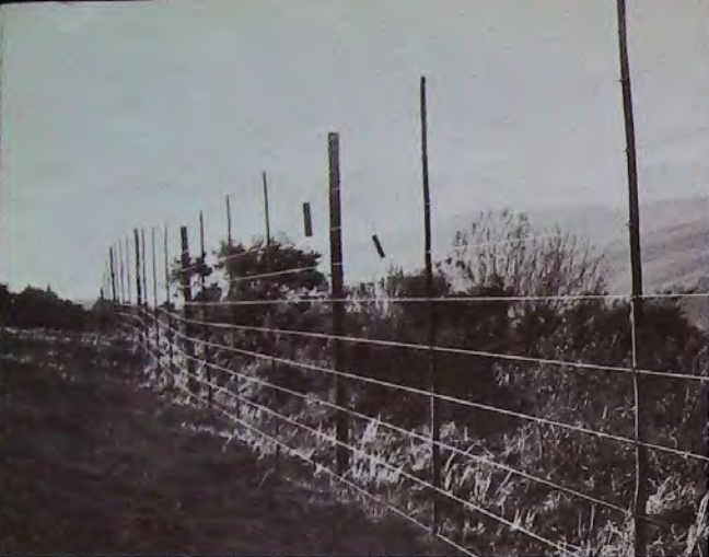
Above: Part of the high game fence being erected around the extension to the Eland Sanctuary. Comprising 10 strands of high-tensile steel wire, the fence is 11 kilometres long and has been paid for entirely from a donation made by the Conservation Trust. Below: The extension to the sanctuary also includes heavily forested areas which will ensure sufficient browse for the national wild herd at Melsetter.
