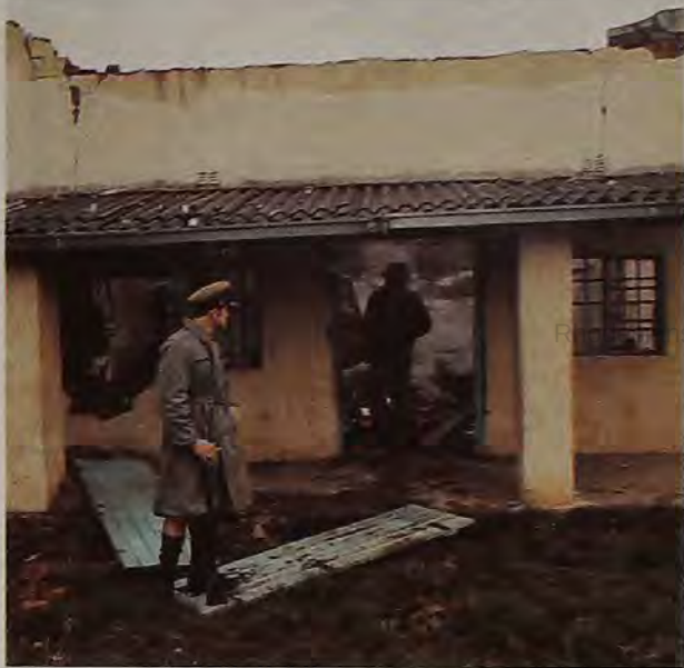
ABOVE: Security Force personnel examine the ruins of an African trading store rocketed by terrorists in the mountain country south of Chipinga.
