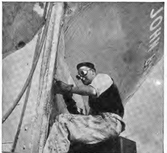
The bow of the John Biscoe has been specially reinforced to make easier going through the iceflows encountered in the Antarctic. This workman is chivelling down the newly reinforced bow after additional metal has been welded on.
