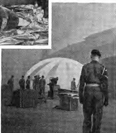
The Portobel being erected in bad weather. It can be used in high winds and is quite stable. Recently, in Belgium, it withstood a 75 m.p.h. wind.
